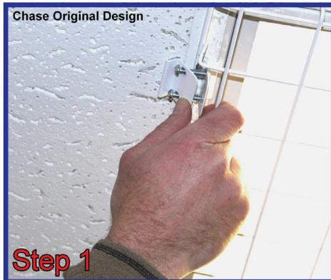
*Be sure to insert the clip with the screw heads facing outside to allow for easy access.*
