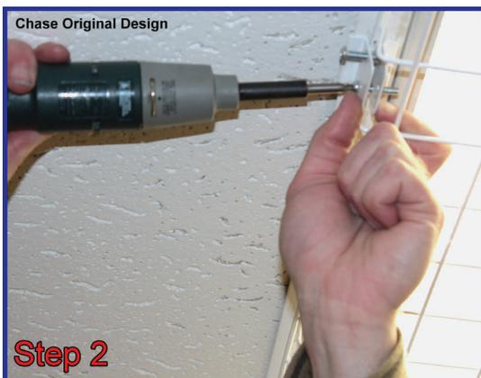
*Draw screws in until the clips meet against the plastic spacers. Do not over-torque as it will cause the clips to bend.*
