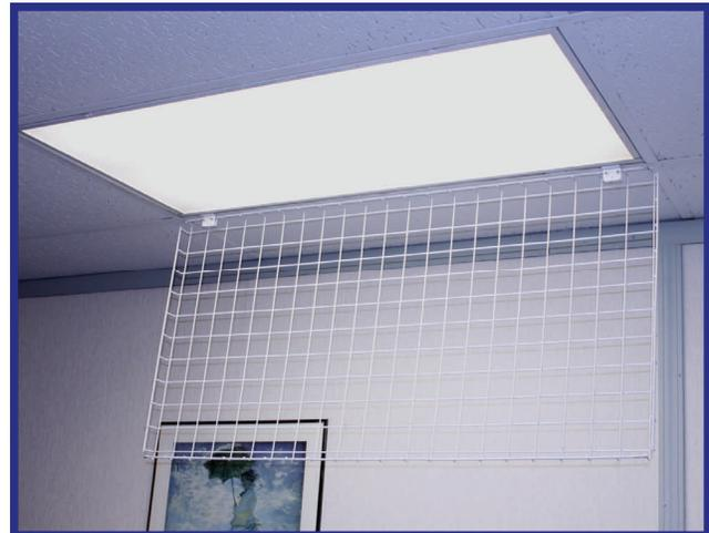
*Leave one side of clips in place to support the unit for routine servicing.*
